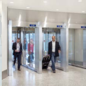
Exit lane breach control
