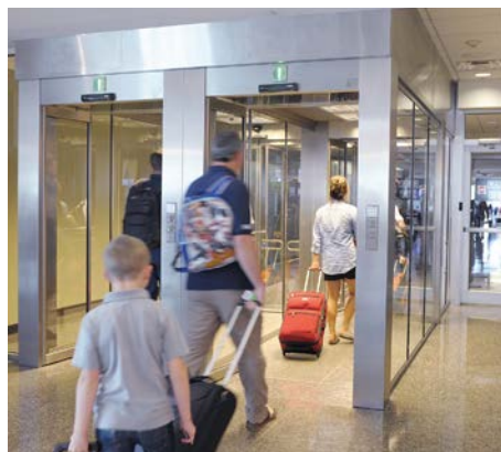
One-way corridors provide unrestricted egress to guide passengers from the airside to the landside.
