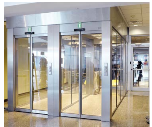
Attempts to enter the airside are detected by sensors and video analytics. Doors are closed and the attempted breach is reported to airport security.
