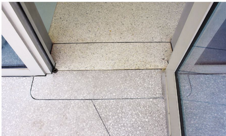
In this opening, the anchors for a welded, marine-grade stainless steel floor strike/receiver are concealed beneath the removable terrazzo cover.
